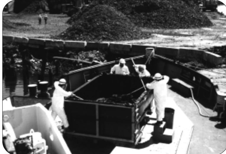
SEDIMENT COLLECTION - NEWTOWN CREEK
